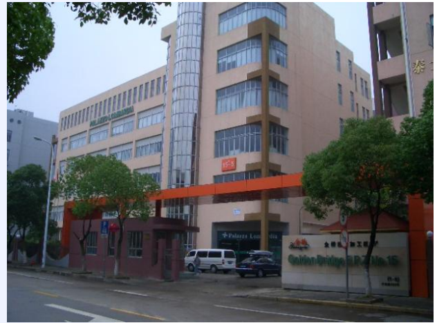
1,500 sqm. manufacturing site in Shanghai
